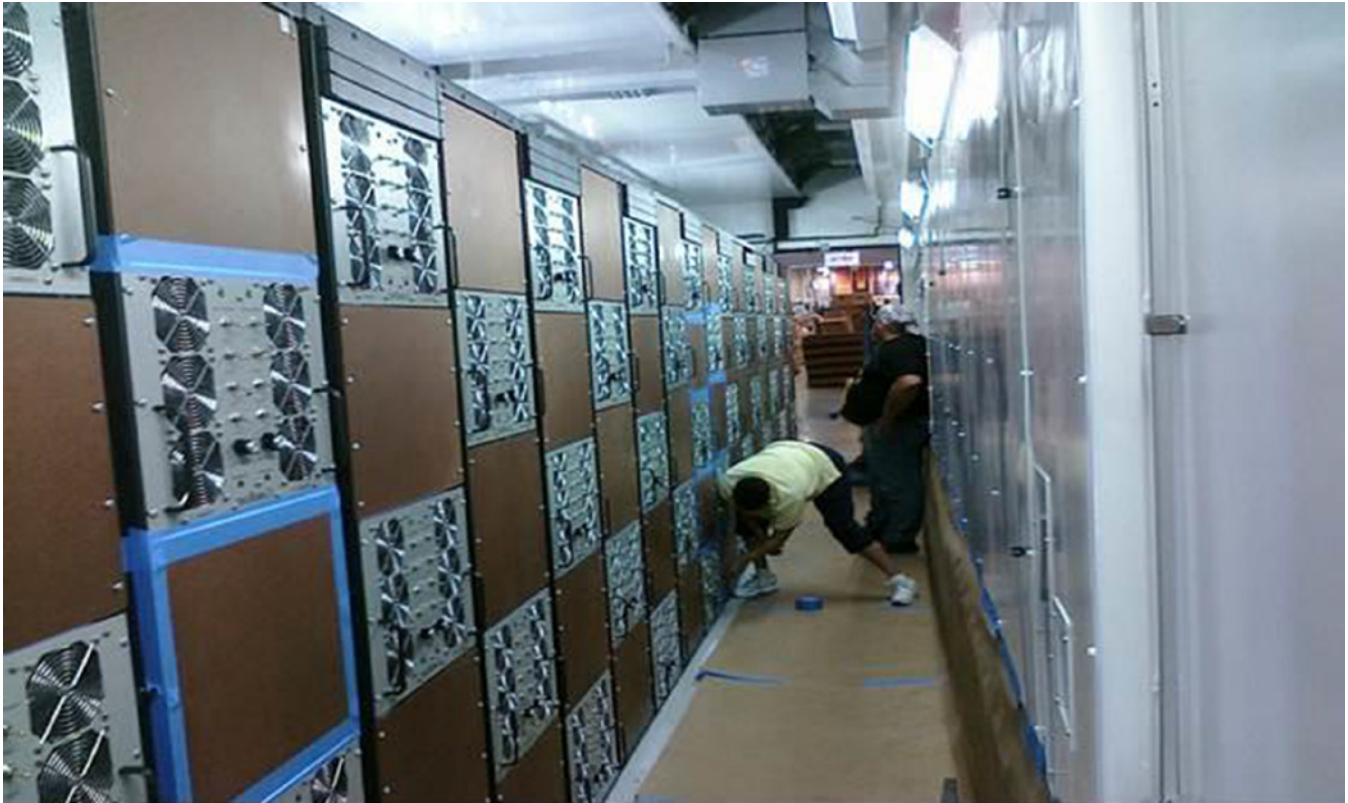
FIGURE 4.24 Test the load with load banks that mimic server sealing and airflow. Courtesy of Hewlett-Packard Company.
