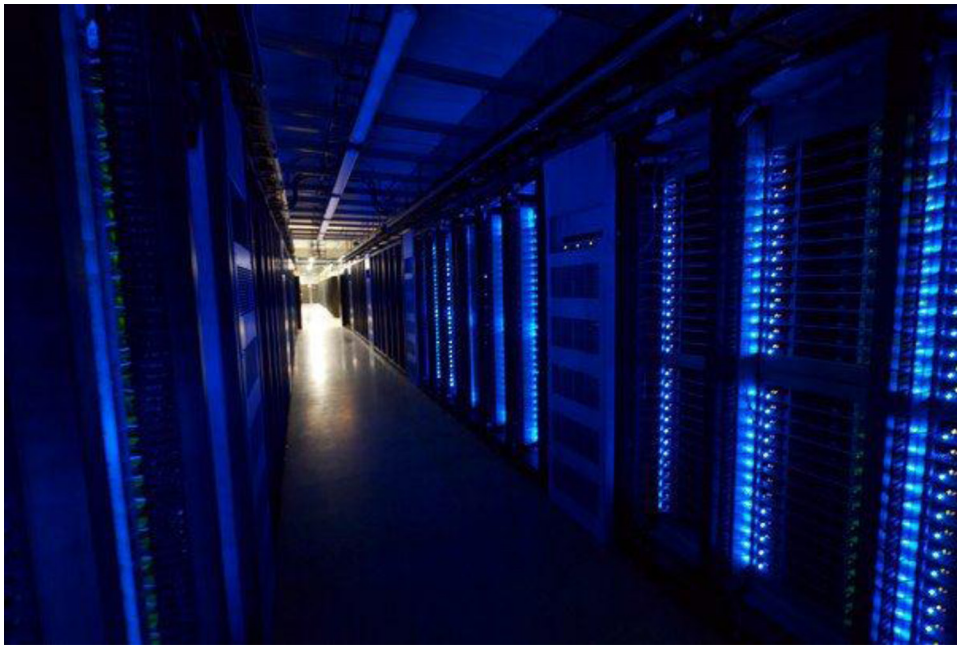
FIGURE 11.9 Facebook data center aisle.
