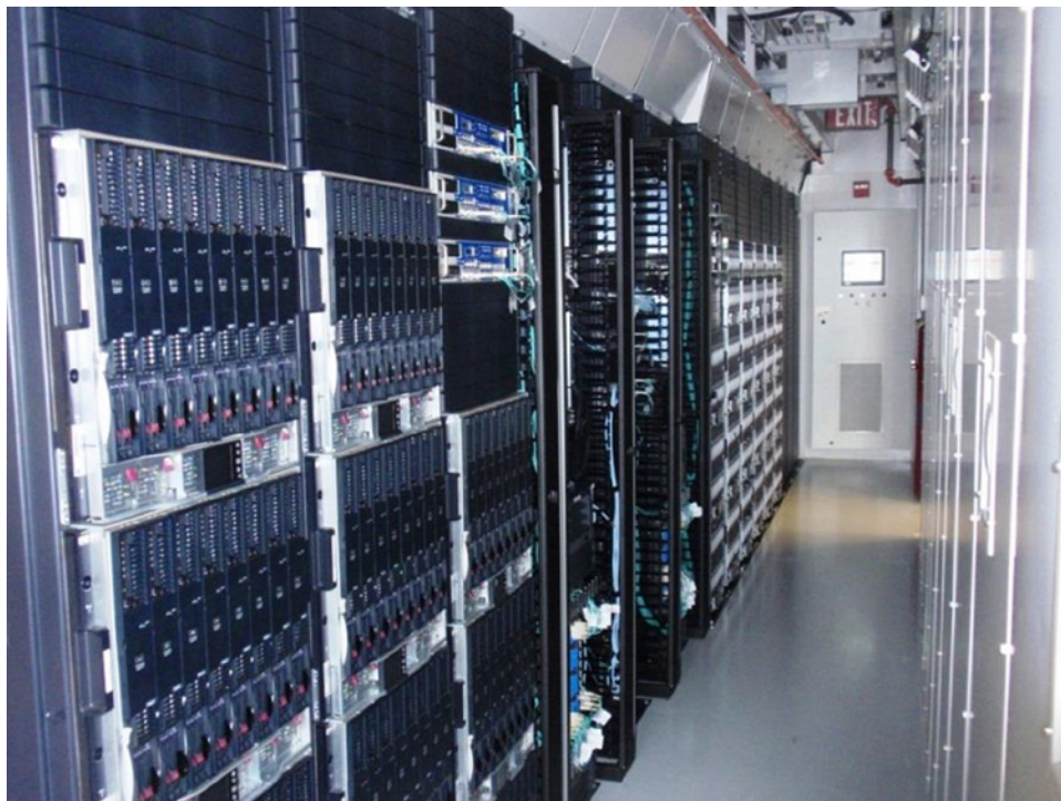
FIGURE 4.16 Having network cabling racks in a few locations can make complex cabling on-site easier at the trade-off of less racks. Courtesy of Hewlett-Packard Company.
