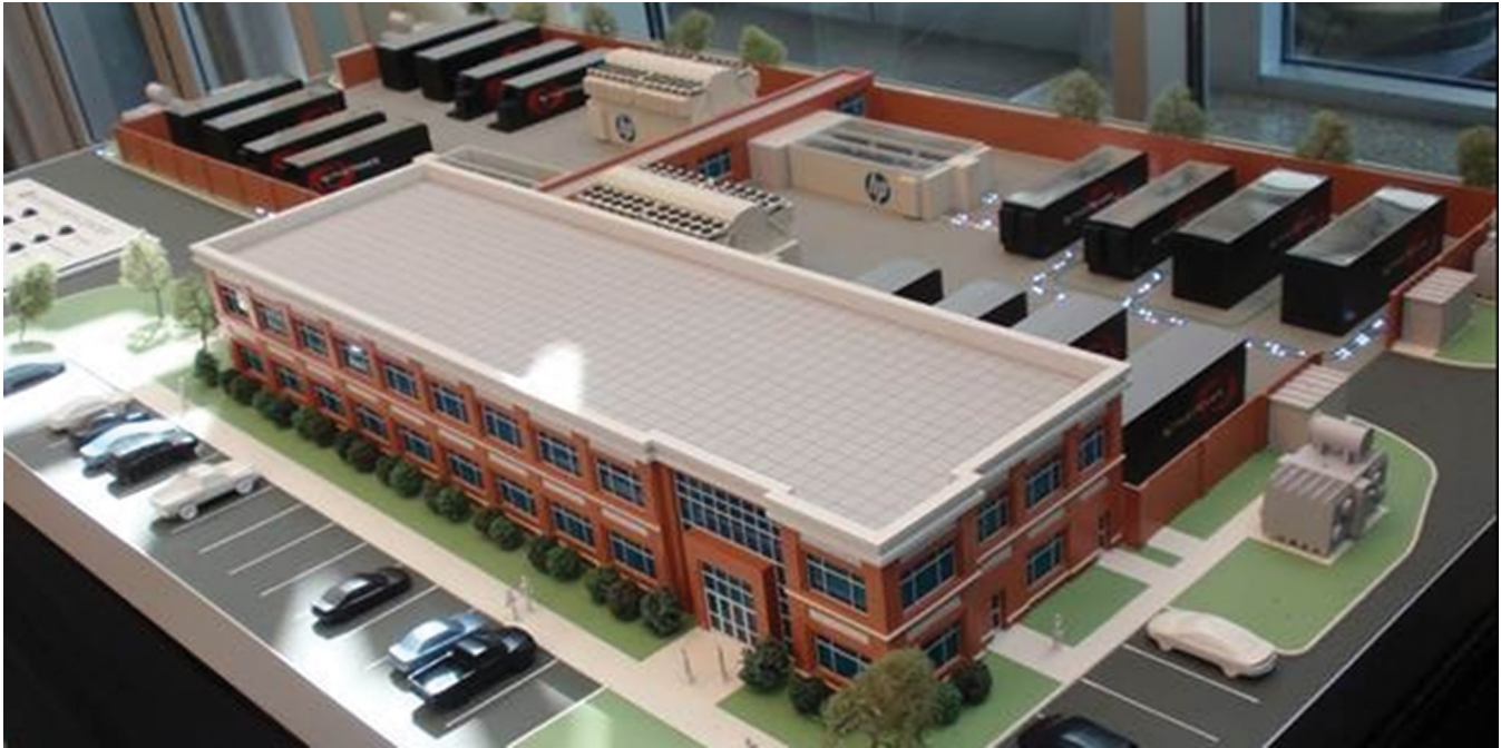
FIGURE 4.1 Example of an MDC. Each of the white and black boxes behind the office space is a manufactured module, and some are totally preassembled. Any one white IT module with its integrated cooling is powered by the four black modules, providing continuous redundant power. That row of five boxes is one 500–1000 kW complete MDC. Courtesy of Hewlett-Packard Company.
