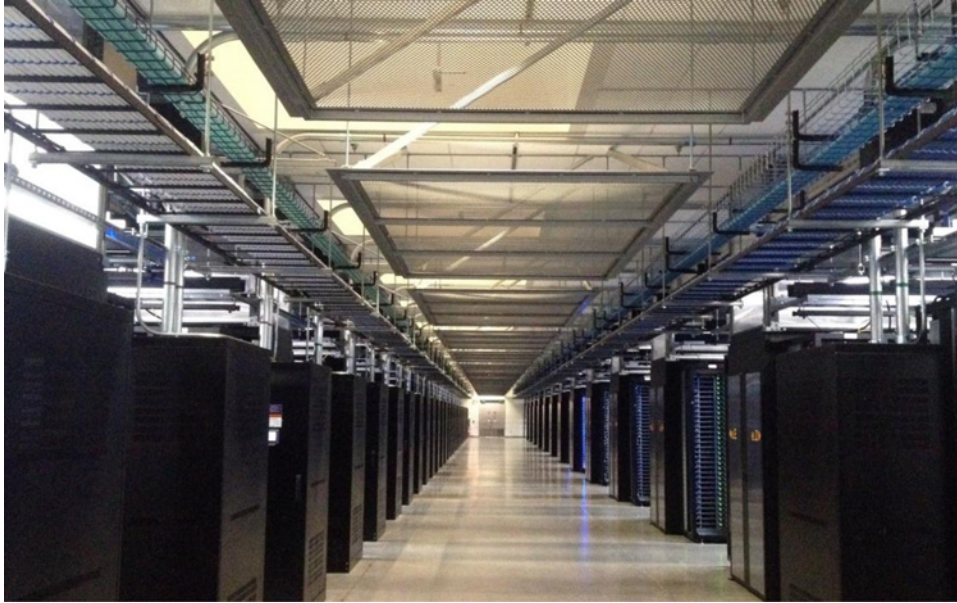
FIGURE 11.8 Facebook data center suite.
