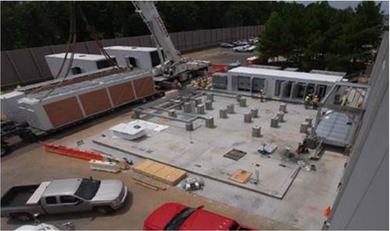
FIGURE 4.20 Tight clearances for long heavy MDC components all arriving at the same time requires complex engineering and planning. Courtesy of Hewlett-Packard Company.
