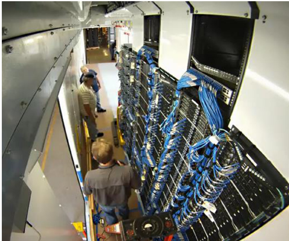
FIGURE 4.12 Front-cabled racks being installed in an MDC at IT factory. Courtesy of Hewlett-Packard Company.
