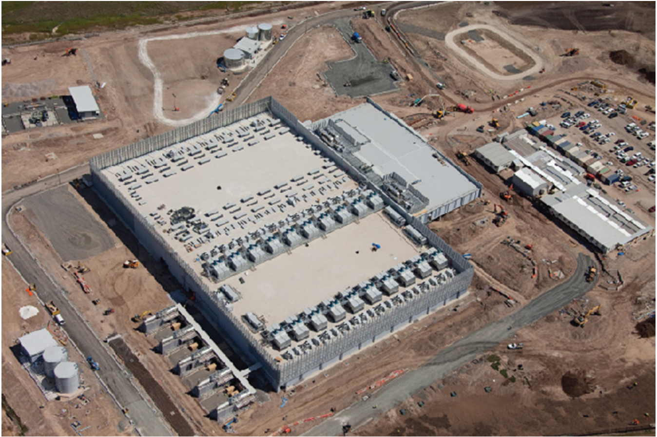
FIGURE 25.11 Aerial view of (42) indirect air-side economizers (IASEs).
