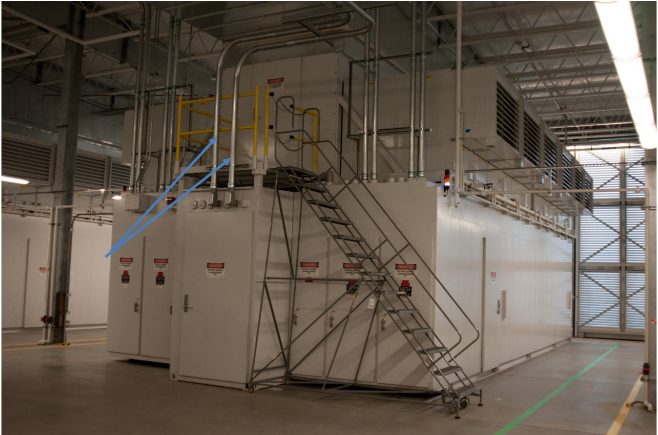
FIGURE 4.17 Adiabatically cooled MDC in a warehouse with the network, control and power conduit connected to the outside world. The two large pipes in the hot aisle extension are a conduit pass through to run the network straight to the site IDF. Courtesy of Hewlett-Packard Company.
