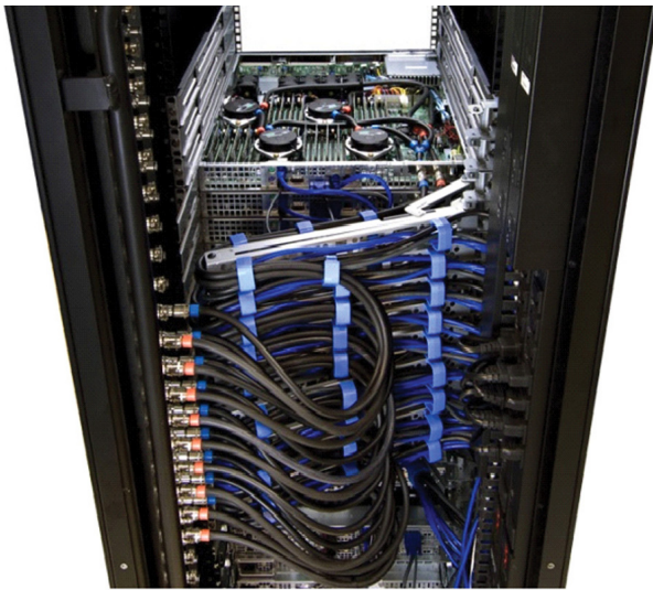
FIGURE 26.10 Water pipes and manifolds. Courtesy of Asetek.
