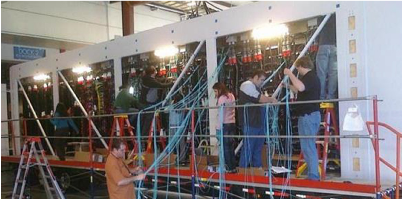
FIGURE 4.15 Complex IT wiring could be much faster in an MDC factory environment. Courtesy of Hewlett-Packard Company.
