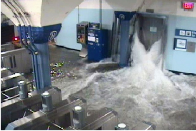
FIGURE 36.5 A subway station in Hoboken, NJ, as well as many in Manhattan, was flooded. Courtesy AP/Port Authority of New York and New Jersey.
