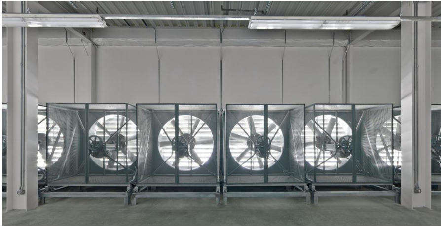
FIGURE 18.8 Relief fans in exhaust corridor. Courtesy of Facebook.
