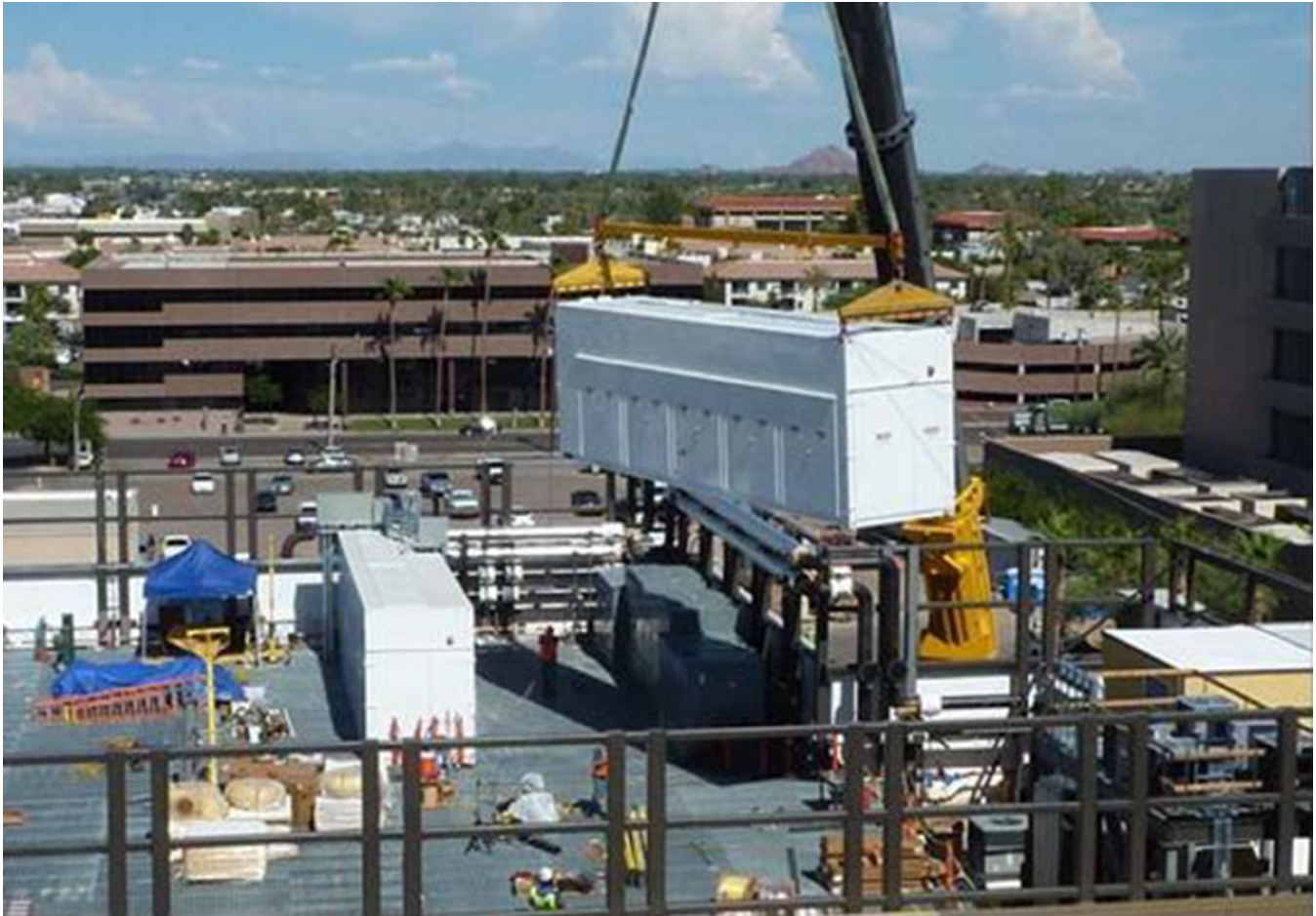
FIGURE 4.21 Not uncommon for MDCs is to scale over time. The first water-cooled container IT is being commissioned, while the second one is being delivered.
