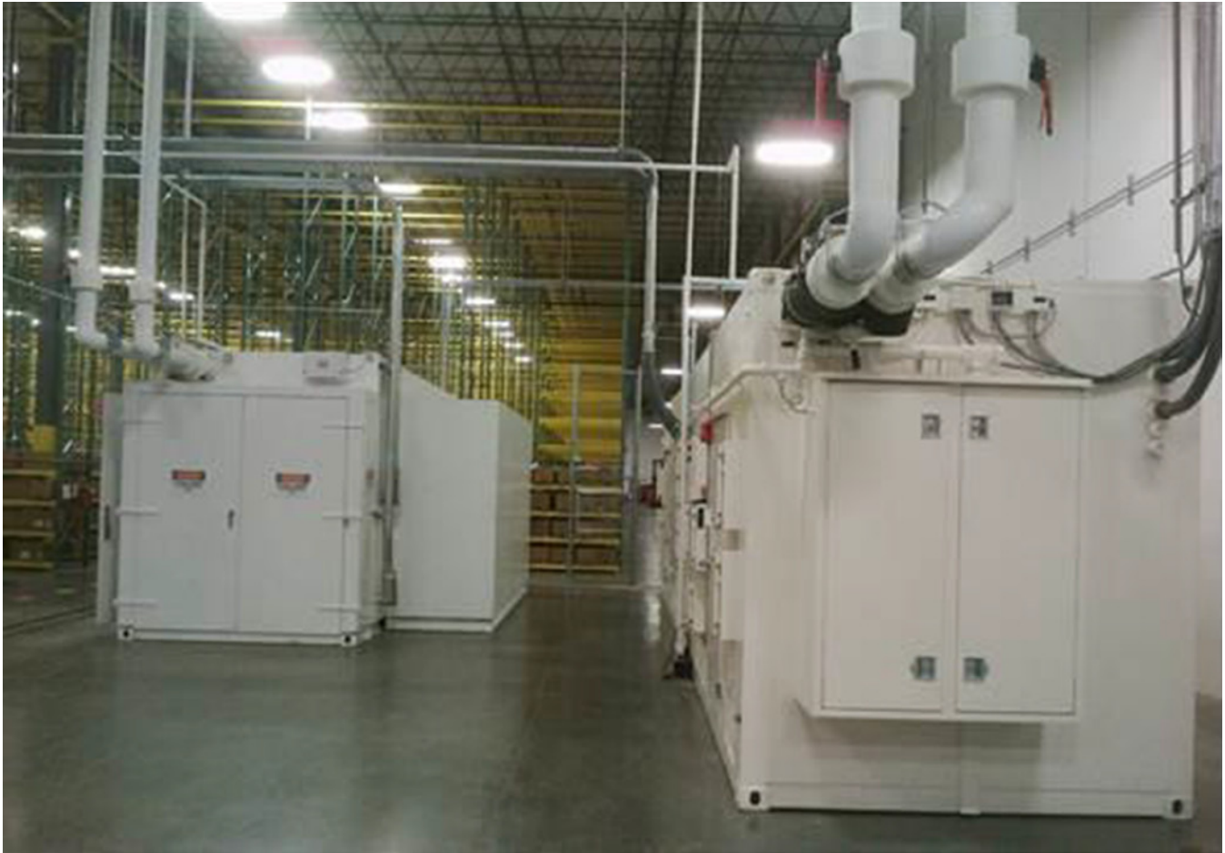
FIGURE 4.22 20-ft water-cooled custom module next to 40 ft standard module. Courtesy of Hewlett-Packard Company.
