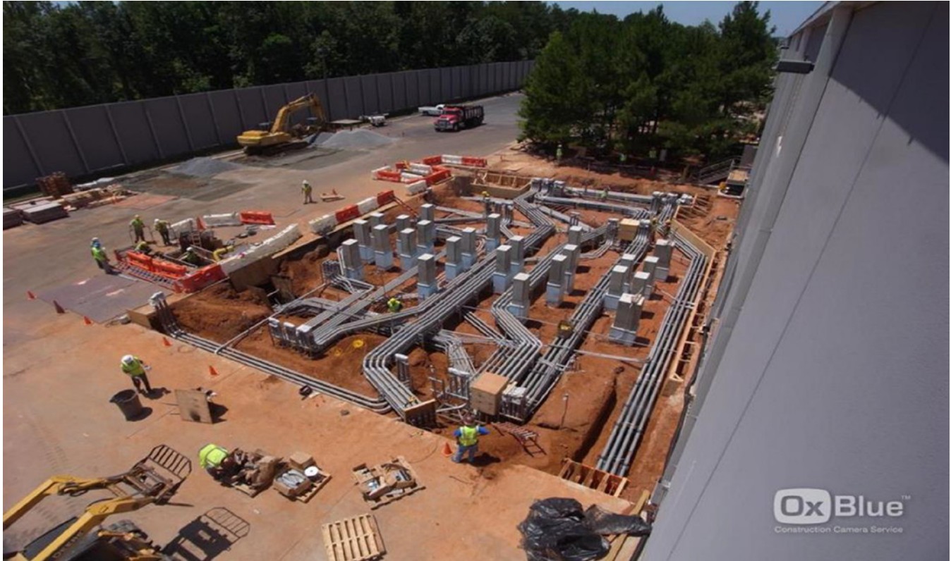
FIGURE 4.19 It takes about 30 days to dig a hole and prep 2.5 MW of electrical conduit to prepare to pour concrete for a 2N 700 kW MDC expansion to an existing data center. Courtesy of Hewlett-Packard Company.
