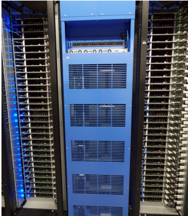
FIGURE 11.10 Facebook DC UPS battery cabinet.
