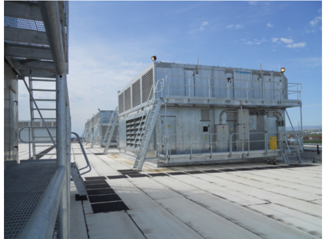
FIGURE 25.8 160,000 cfm IASEs with heat wheels removing a total of 10mW of heat from a data center.
